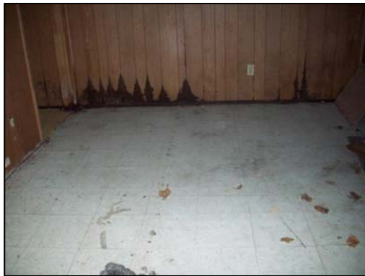
12" Floor Tile with Streaks Basement
