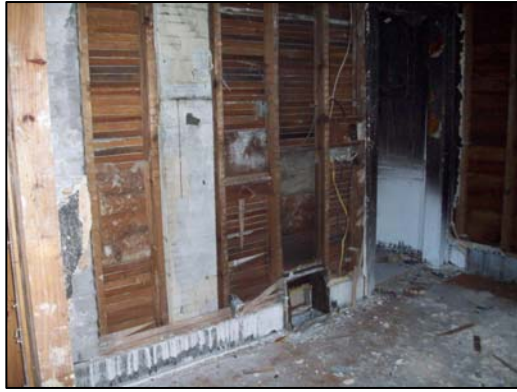
Duct Wrap Register Boots/Runs Throughout
