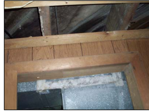
Duct Wrap – 2" Tape Basement
