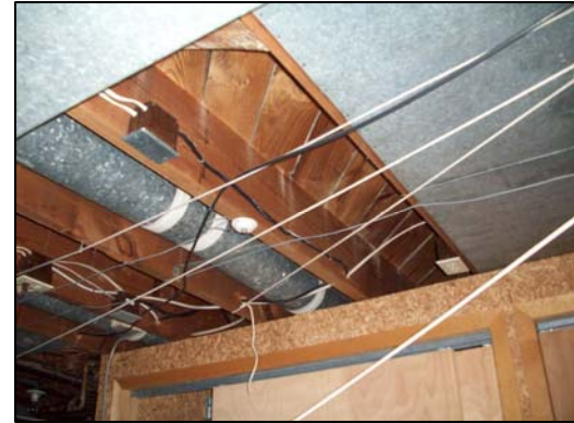
Example of Duct Wrap – Basement FRIABLE
