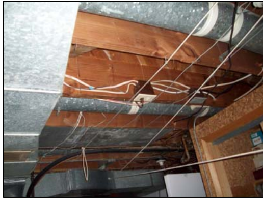
Example of Duct Wrap 2" Tape – Basement FRIABLE
