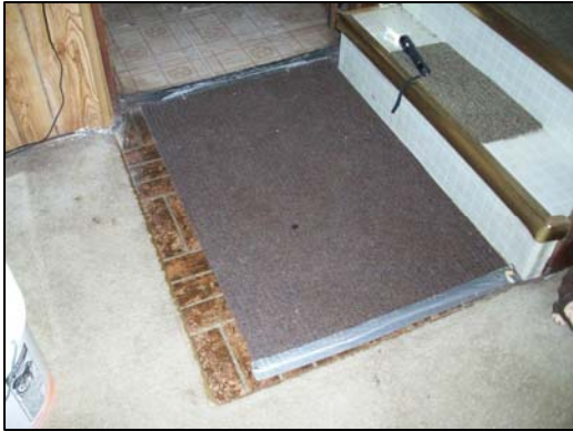
Floor Tile beneath Brown Linoleum – Bottom of Basement Stairs NON FRIABLE
