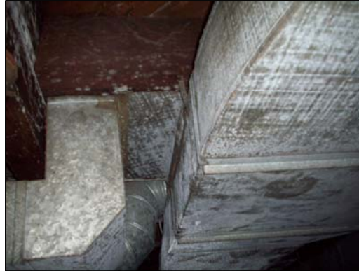
Example of Duct Wrap Basement
