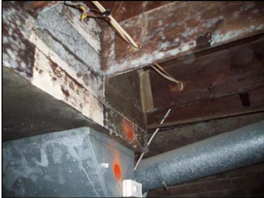
Example of Duct Wrap Basement
