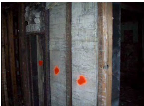
Example of Duct Wrap Insulation 1 st Floor Apartment/Basement
