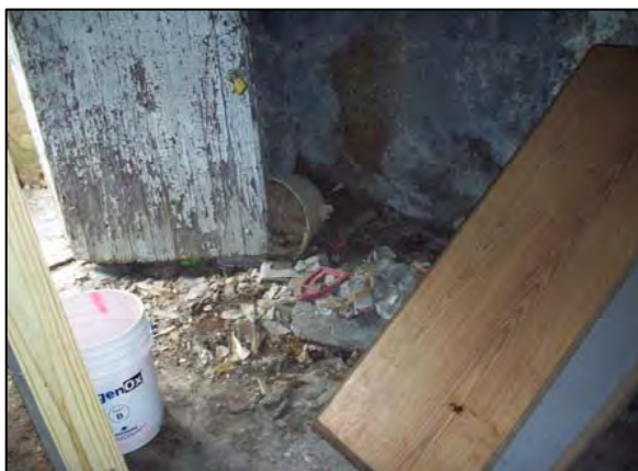
Example of Debris Piles with Duct Wrap Insulation Basement
