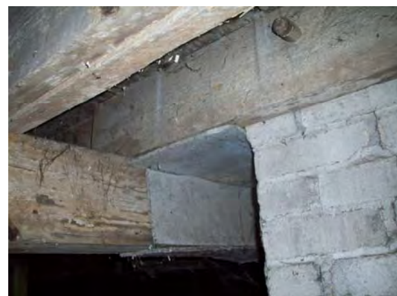
Example of Fire Board (Transite) Basement
