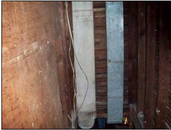
Duct Wrap Boots and Runs Throughout
