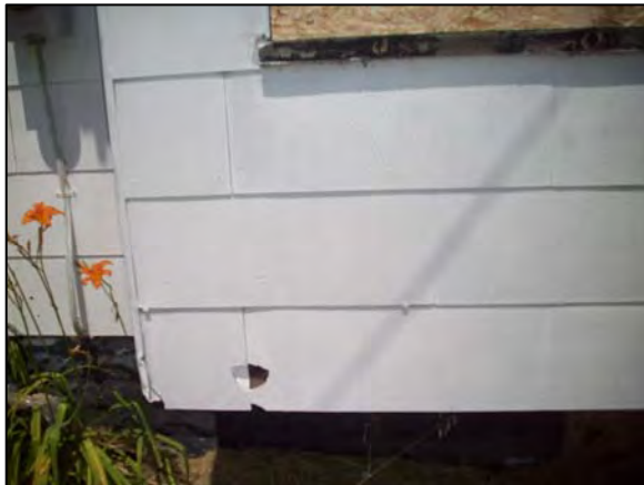
Transite Exterior Siding
