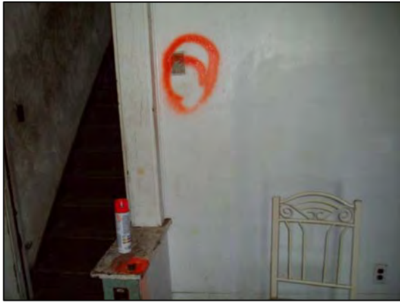
Smoke Detector and Thermostat Living Room
