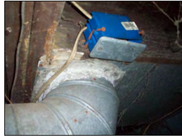
Duct Wrap Basement
