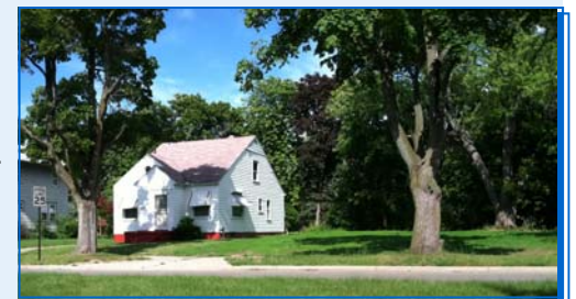
Above: Photo of residents home next to a recently demolished home in Civic Park.
